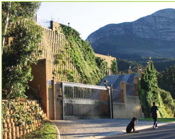
HEAVY GRAVITY RETAINING 7M HIGH
