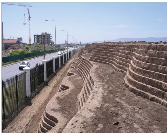
MEANDERING TERRACES FOR NOISE BARRIER
