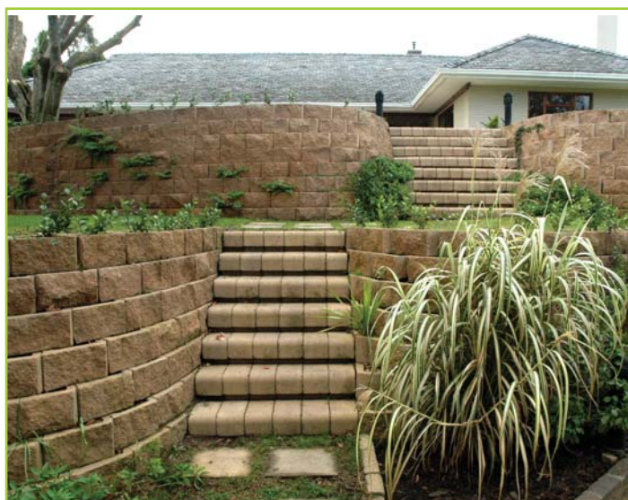
DECORATIVE ROCK FACE GARDEN WALL AND ACCESS STAIRS
